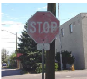
A faded, non-reflective, and graffiti covered "STOP" sign that needed to be replaced
