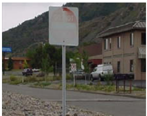
A faded and non-reflective "DO NOT ENTER" sign that needed to be replaced
