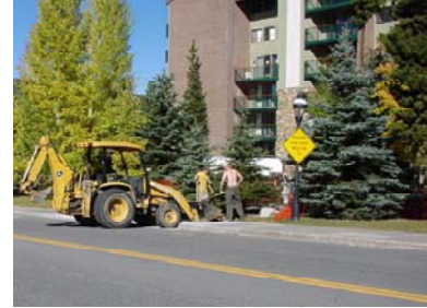
Excercising control over work occuring within your right of way
