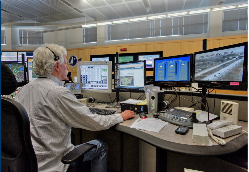
MN Department of Transportation
