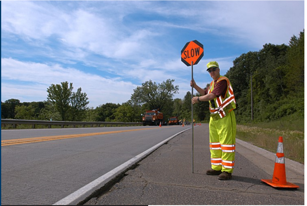
MN Department of Transportation
