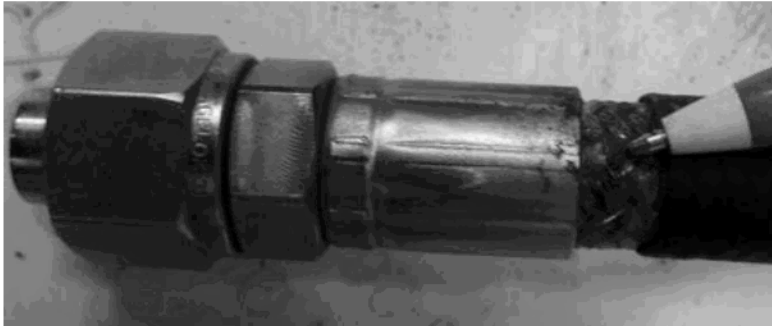
Figure 3 Corrosion at the braid and fitting. A pen shows where a leak is located.
