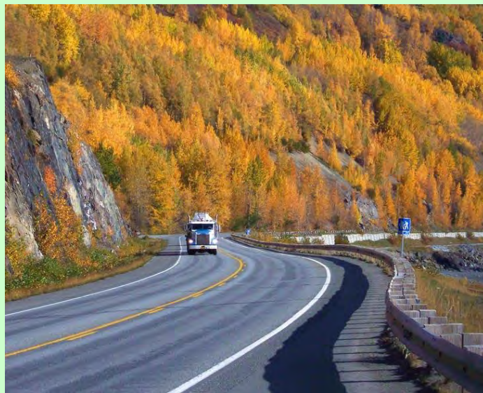
Seward Highway (MP 110). Photo by Jack Stickel, Alaska DOT&PF
