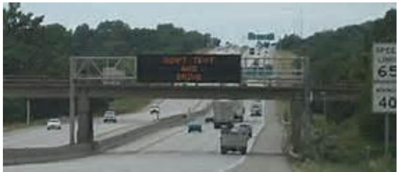
The state of Iowa now utilizes the Iowa Department of Transportation's dynamic message boards to display traffic safety messages.
