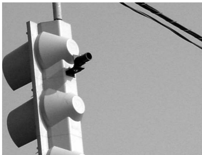
The "rat box," shown attached to this traffic signal, indicates when a traffic signal is red, allowing an officer to be downstream of potential offenders.
